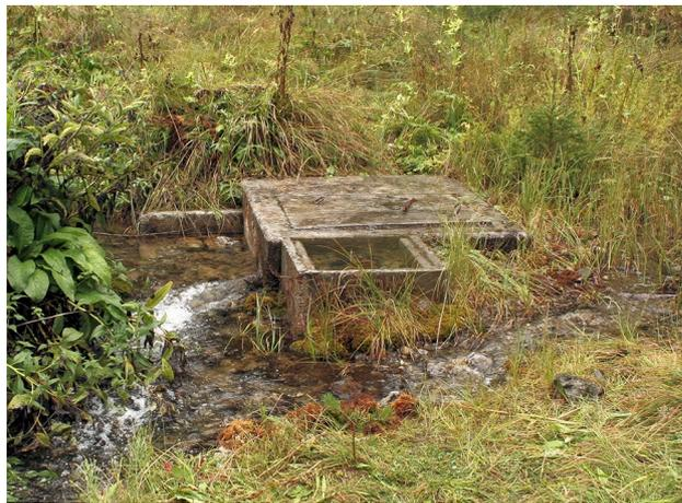
**Figure 8.** Springs of the Dorfbach. Historically, the water was used as Biberwier's drinking water supply. The concrete structure captures the middle of the three springs, the other two coming from the left and the right to the structure (image taken 2007-09-06).
