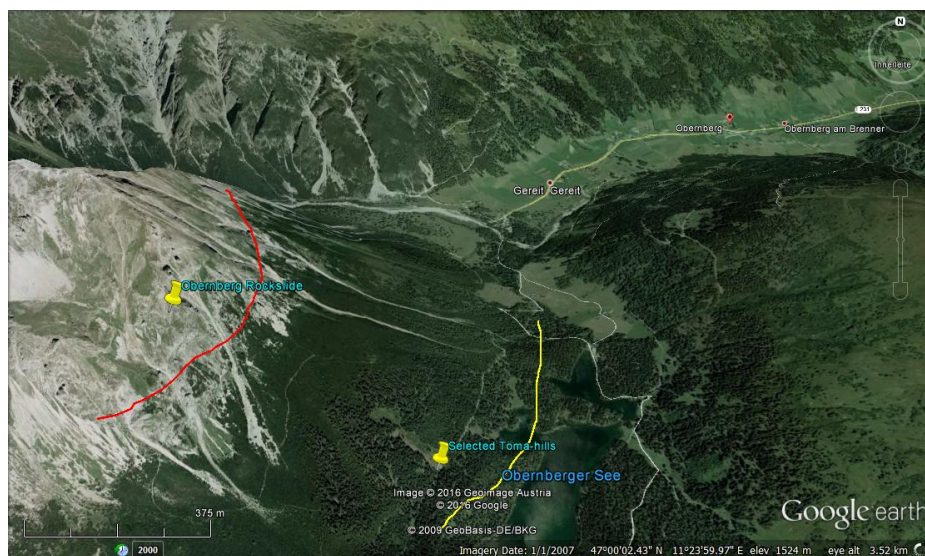
Figure 3.6: Obernberg rockslide location (© Google Earth)
